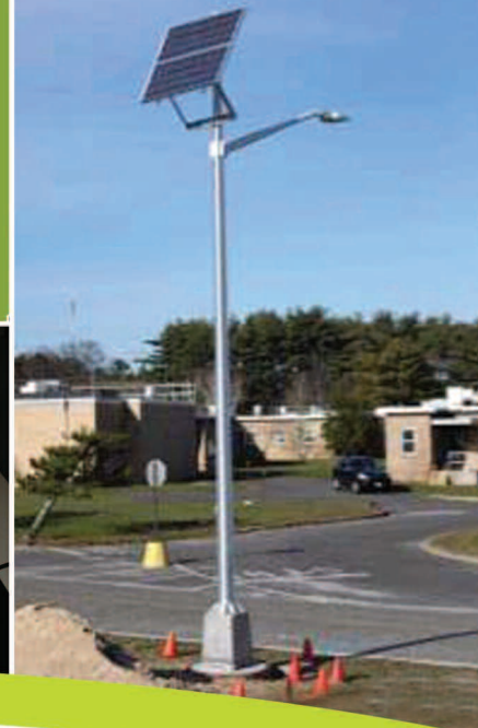
Solar/LED Pole Installation
